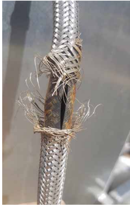
The stainless steel braided sleeve corrodes, causing the rubber inner tube to expand and burst. Image supplied by Neil & Craig Baker Plumbing - NSW.
